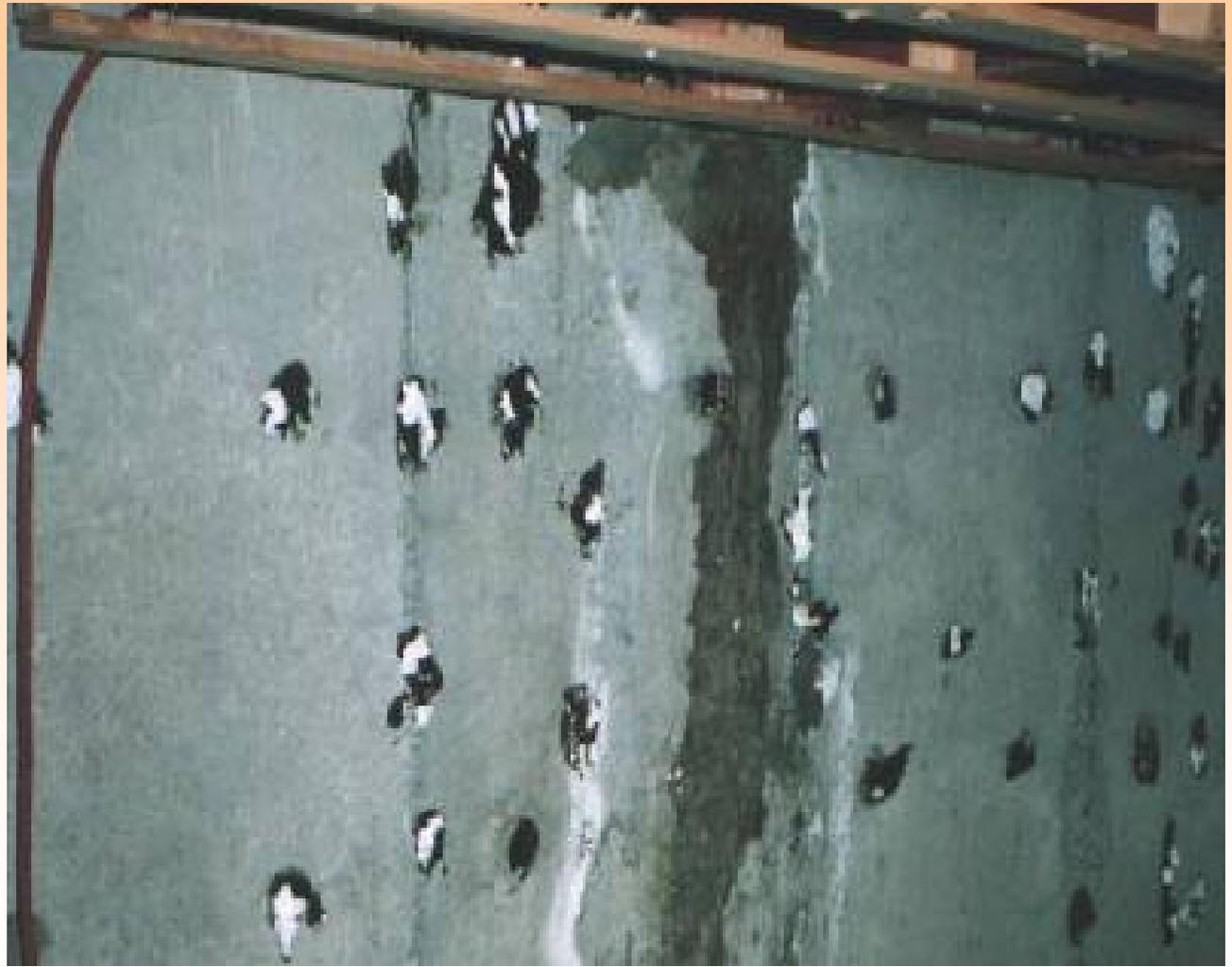
**Mold growth was found in the corners of this basement when the insulation was removed.**
